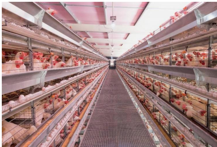
Figure 2: Conventional cage (manure belt) hen house (photo credit: Big Dutchman).
